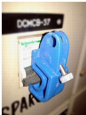
Fig. 6: MCB Lockouts
