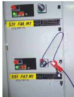
Fig. 10: Cable Lockout
