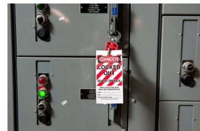
Fig. 8: Feeder Lockouts
